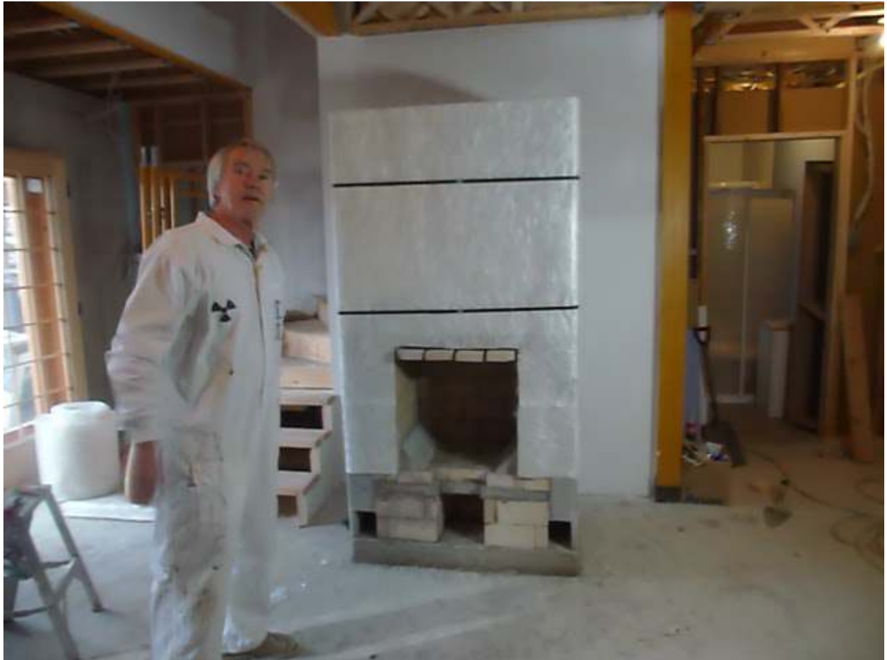
Heater core with fiberglass matt slip joint installed. Ready for facing. This one does not have an oven.
