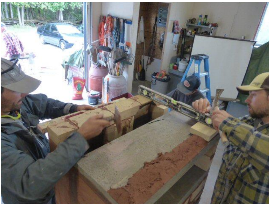
Height adjustment course above the bake oven to bring both sides level.
