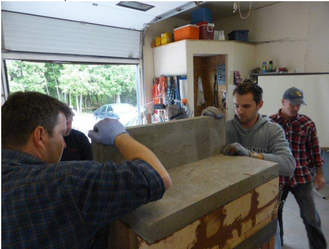
Installing the bake oven back.
