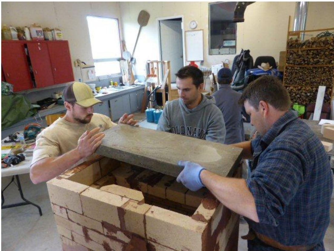
Intstalling the bake oven floor.
