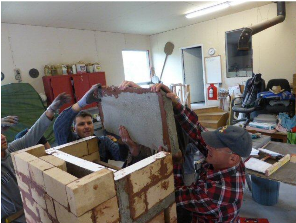
Installing the bake oven ceiling.
