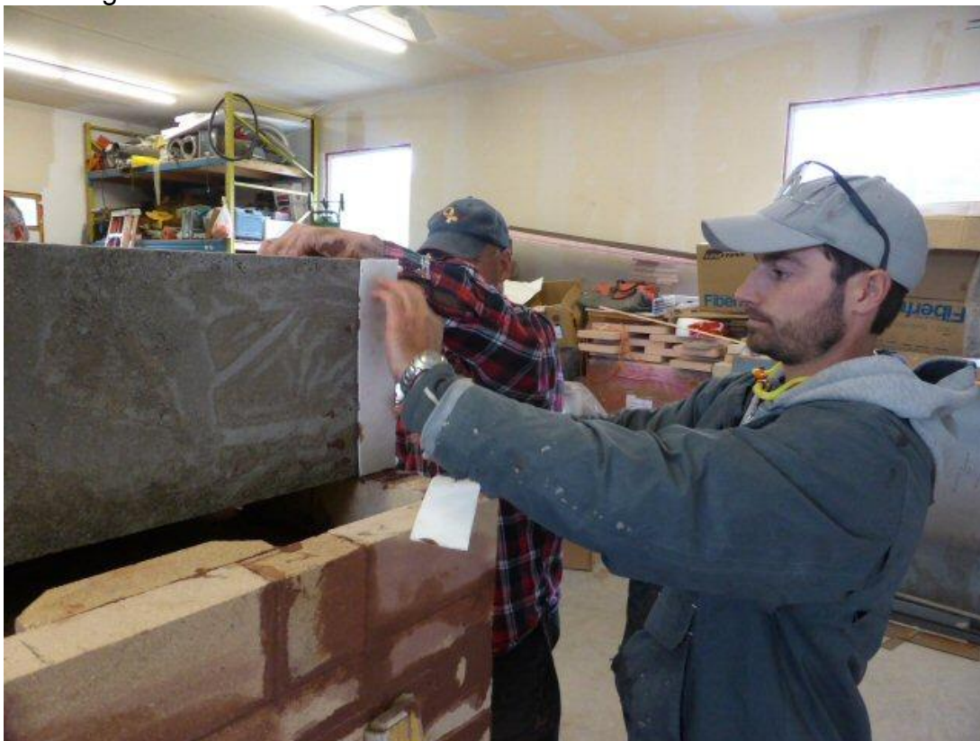
Gasketing the rear of the bake oven rear slab.
