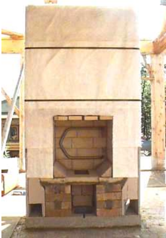
An installed side exit coil.
