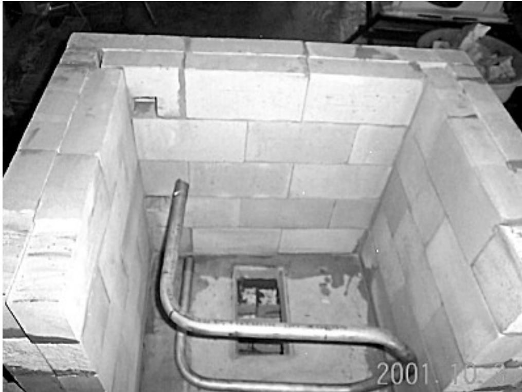
A rear exit coil about to be installed in the firebox.
