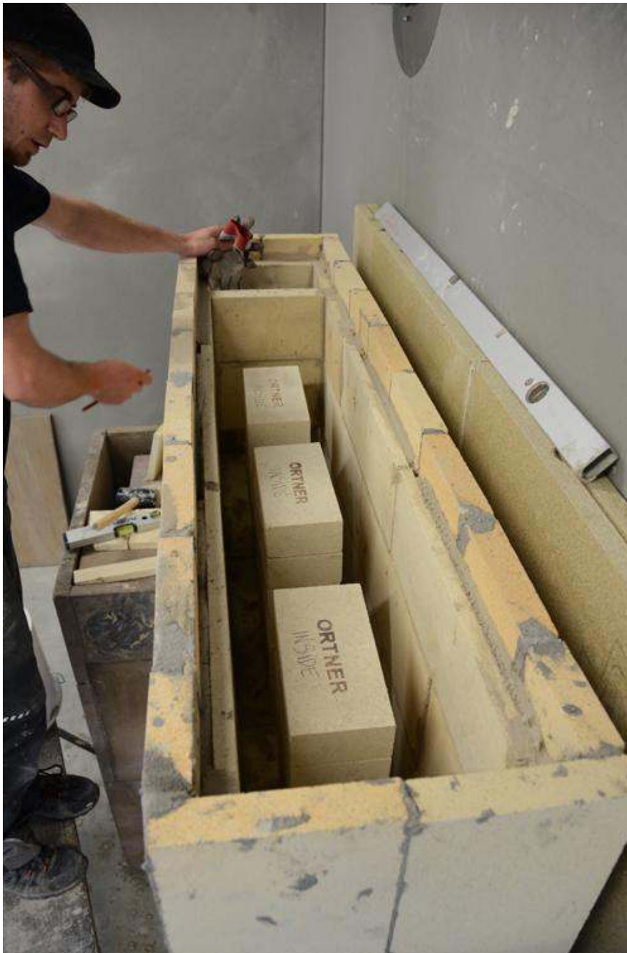
Upper bell. Dry-stacked columns inside. Updraft into the chimney connection at the back.
