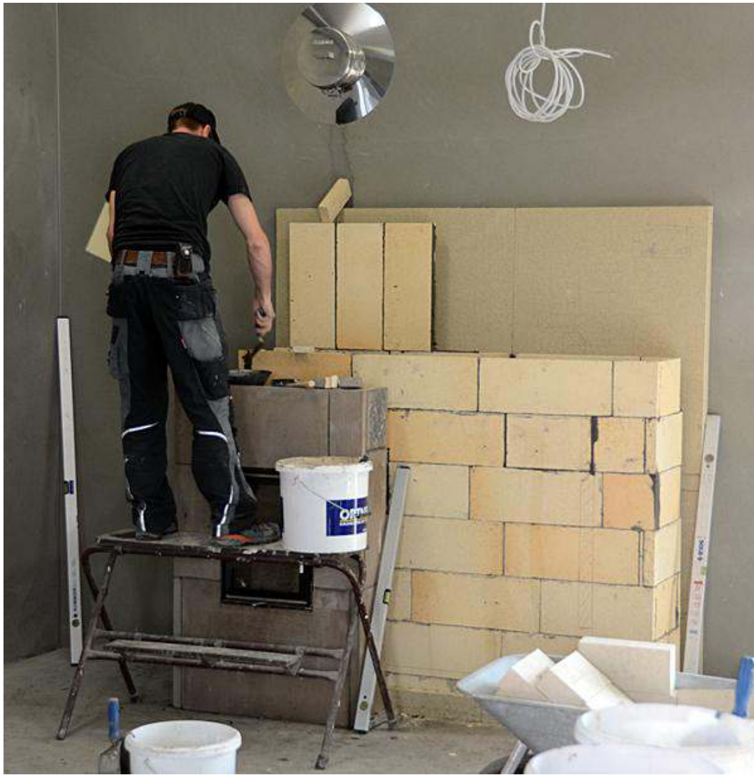
Paul working on the double-bell heater. Note that firebox has facing. No facing on the heat-exchange portion.
